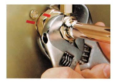
8. After all connections have been made, and after the king valve has been opened (do not open yet), check the couplings for leaks.
