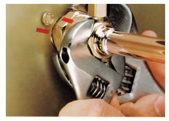
8. After all connections have been made, and after the receiver outlet valve has been opened (do not open yet), check the couplings for leaks.
