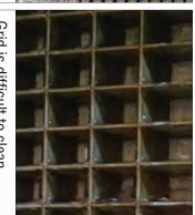
premature equipment failure. diminished production, A dirty evaporator can cause Grid is difficult to clean. increased service cost and
