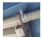
6. Disassemble fixed screws which are in the spray pipe. Dismantle the spray pipe.
